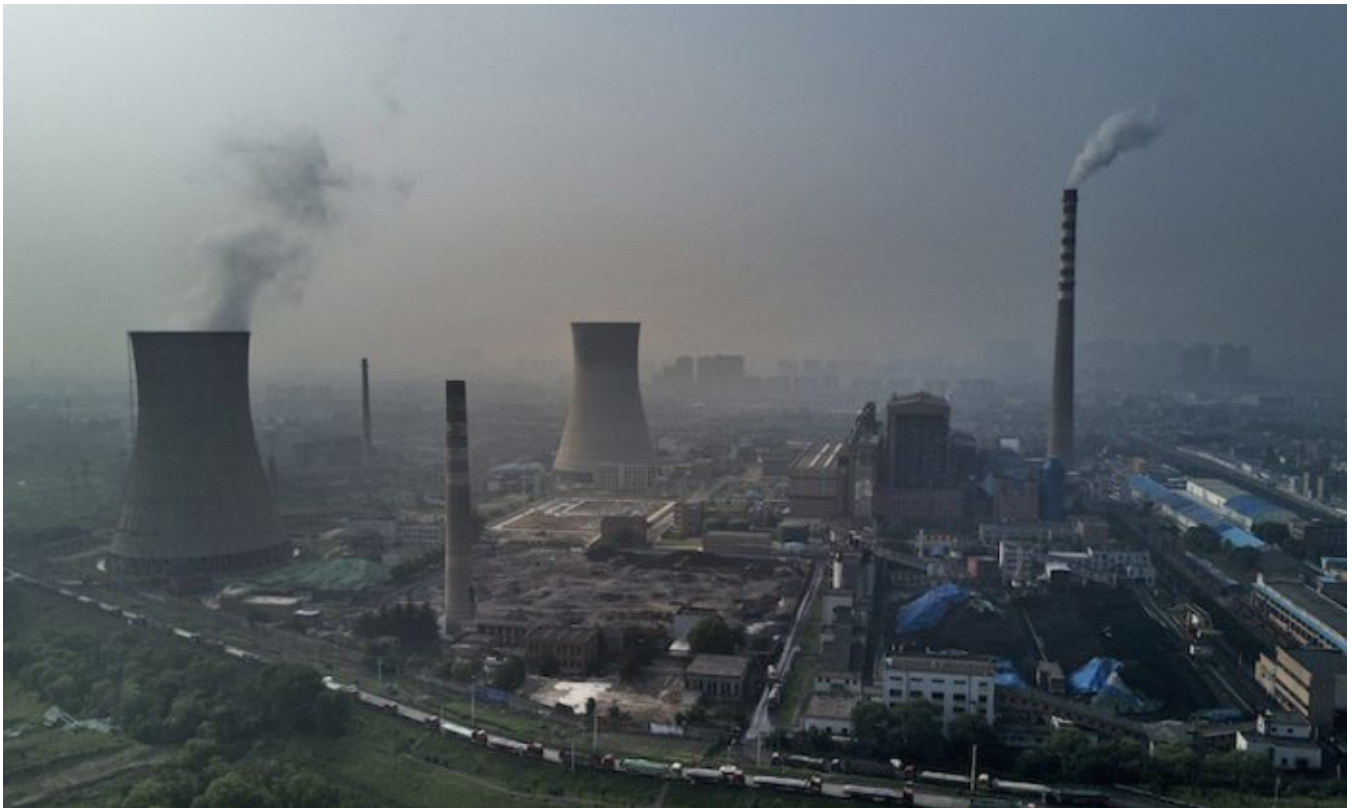
A Chinese state owned coal-fired power plant is seen in Huainan, Anhui province, China, June 16, 2017. (Kevin Frayer/Getty Images)
