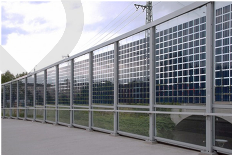
Figure 8-10. Fence/Noise Barrier Solar PV Options
