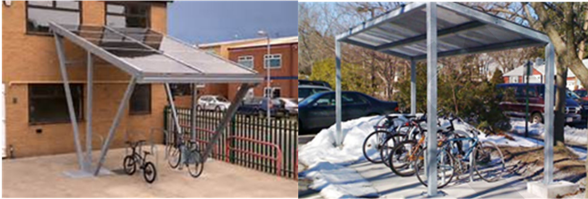
Figure 8-11. Bike Canopy Solar PV Options
