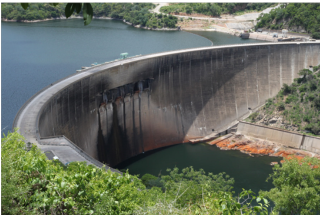
Zimbabwe and neighbouring Zambia heavily rely on hydro-electric power from Kariba Dam.
